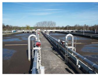
By using the Egger Iris® Diaphragm Control Valves, the oxygen concentration accuracy in the aeration tanks could substantially be improved ( $\pm$  0.1 mg O<sub>2</sub>), which resulted in considerable energy savings.
