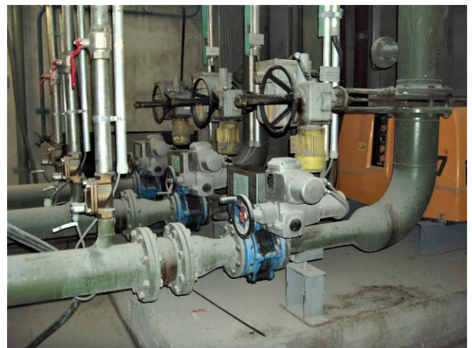
Iris® Diaphragm Control Valves for sludge feeding of the centrifuges in the combined heat –power plant Munich North
