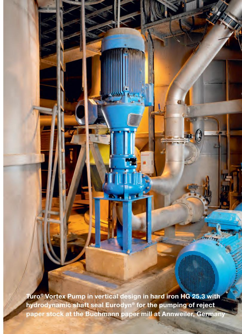
Turo® Vortex Pump in vertical design in hard iron HG 25.3 with hydrodynamic shaft seal Eurodyn® for the pumping of reject paper stock at the Buchmann paper mill at Annweiler, Germany
