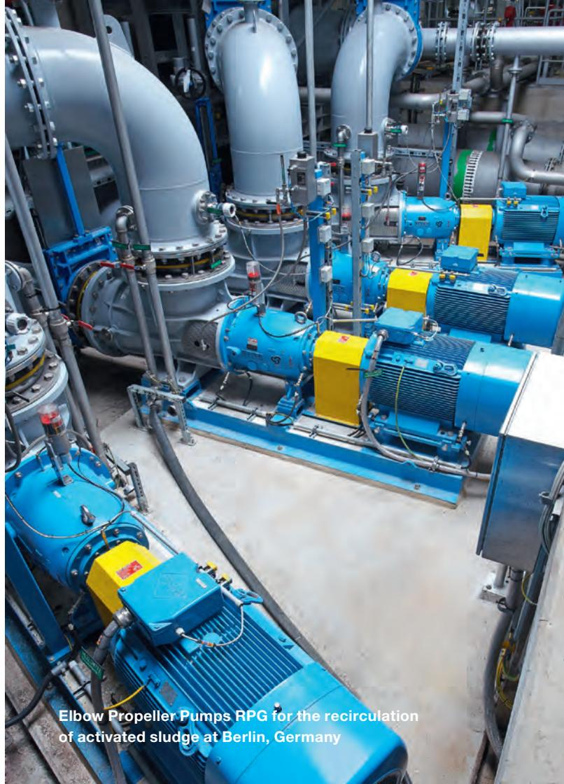
Elbow Propeller Pumps RPG for the recirculation of activated sludge at Berlin, Germany
