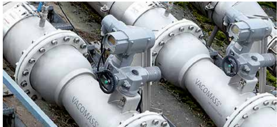
Figure 9 – Binder Vacomass Jet Valve (Courtesy of Binder)
